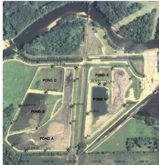
Coal Ash ponds at Eagle Valley.
