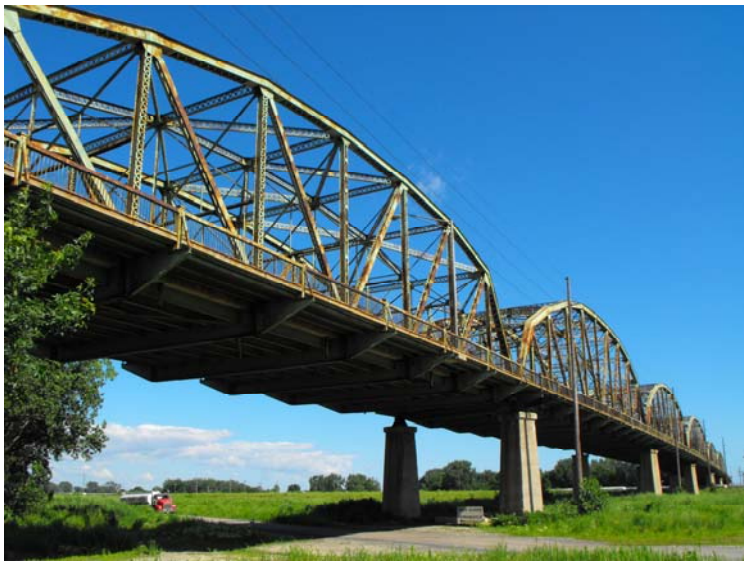
Nine-Span Bridge Hammond
